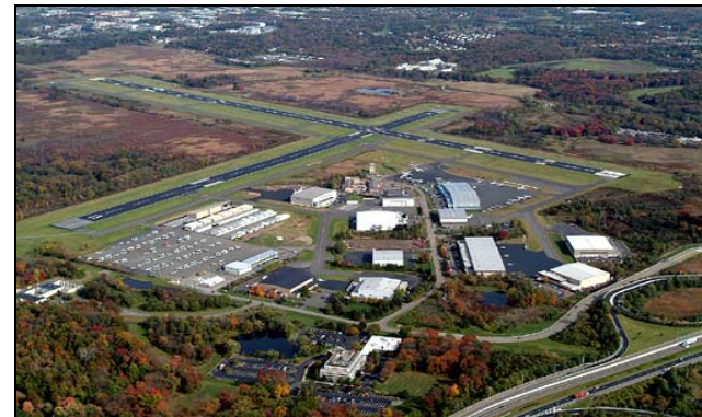
Morristown Municipal Airport
